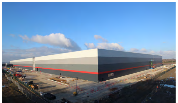
Progress image of Plot 4 SEGRO Logistics Park Northampton
