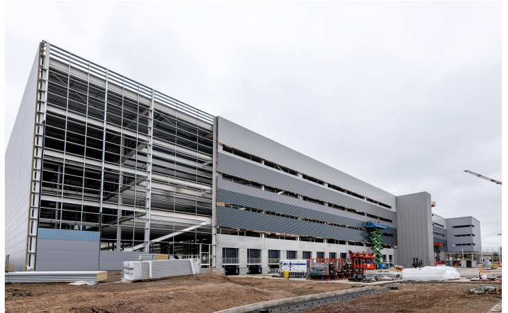
Progress image of Plot 7 SEGRO Logistics Park Northampton
